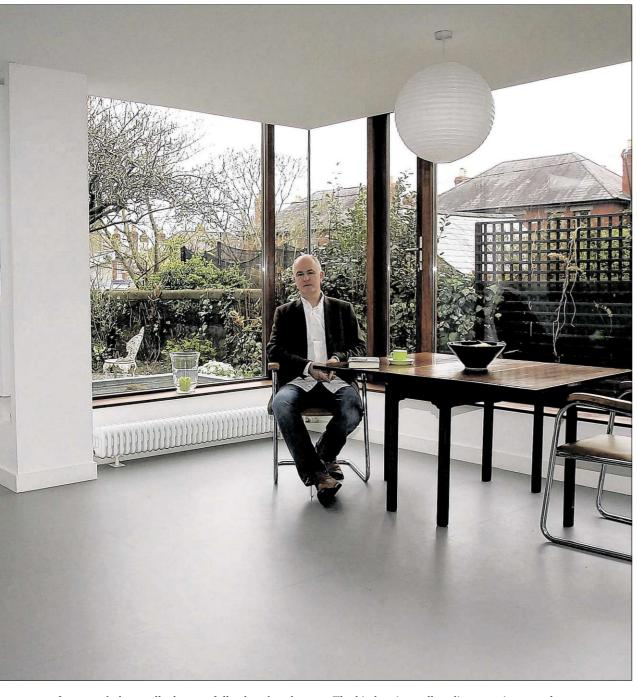
frame and glass walls that are fully glazed at the corners. The glass disappears up past the floating ceiling internally, adding to the feeling of lightness, while outside this allows the zinc roof to be thin.
